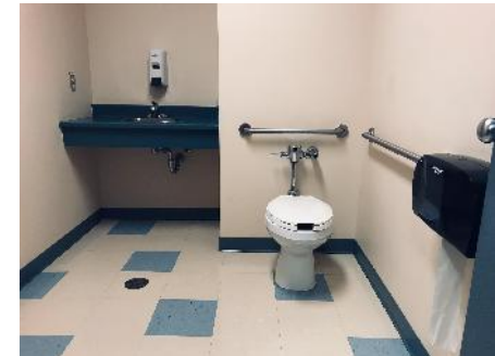
Police Station, Lobby Washrooms
