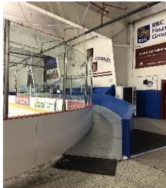
Centennial Arena, Ramp to Separated Accessible Seating
