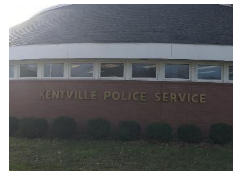
Police Station, Signage
