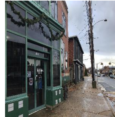
Main Entrance, Kentville Town Hall
