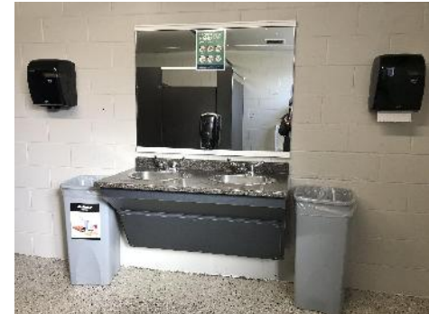
Centennial Arena, Accessible Sink
