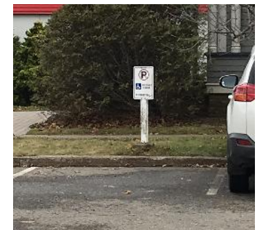
Kentville Library, Accessible Parking does not have safe path to Library entrance
