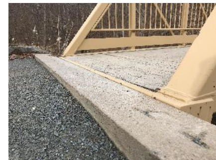
Miner's Marsh, Bridge - Grading Required
