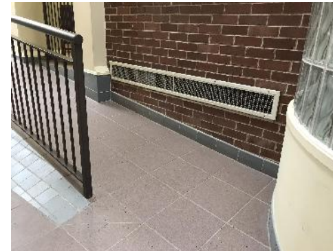
Interior Ramp, Kentville Town Hall
