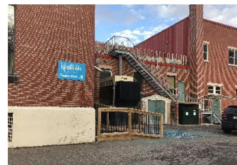
Accessible Parking, Kentville Town Hall
