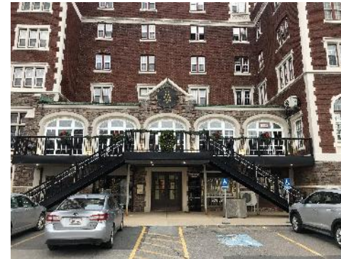
Main Street Station, Parking
