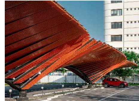
Solar Powered Parking Structures
