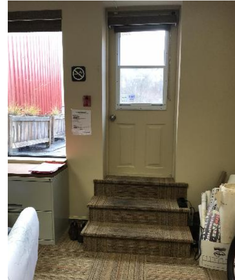
Access to Emergency Exit, Kentville Town Hall
