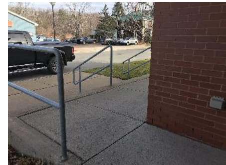
Police Station, Access from Parking Area
