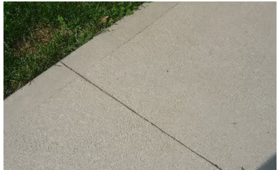
Top Kentville Sidewalk with trowelled joints
