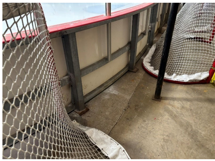
Existing concrete slab with construction joint along boards
