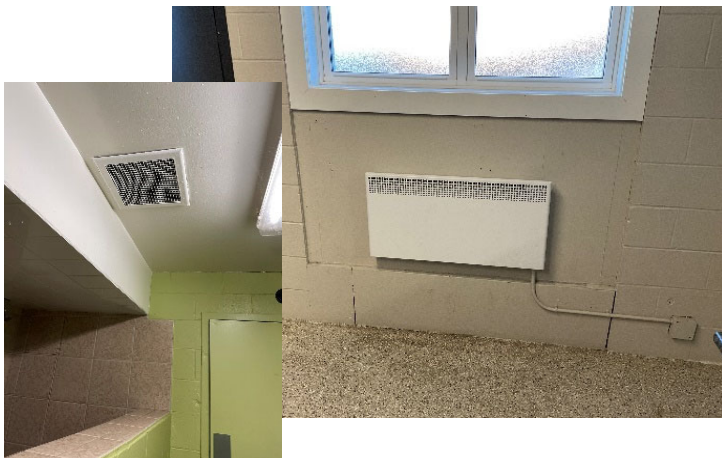
Diffuser from Indoor Evaporator
