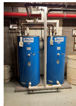
Heat Recover Hot Water Storage Tanks
