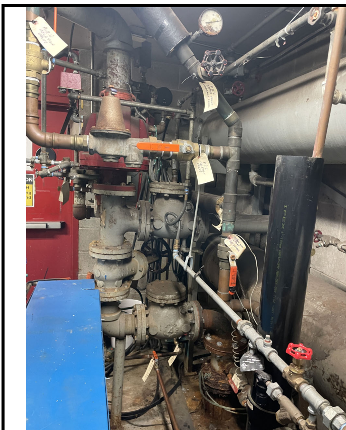
Water service entry to mechanical room
