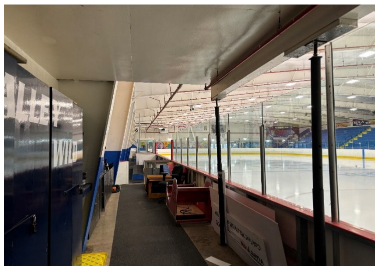
View of mezzanine structure including beams and jack posts
