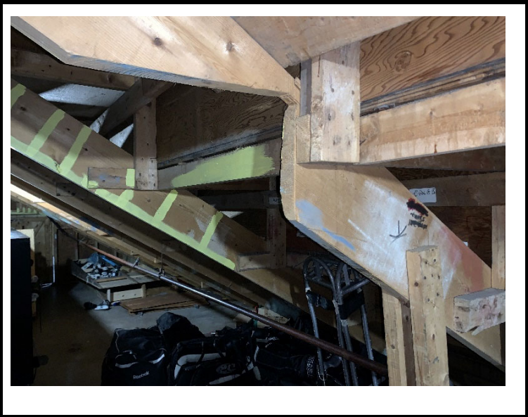
Notches cut into beams under bleachers
