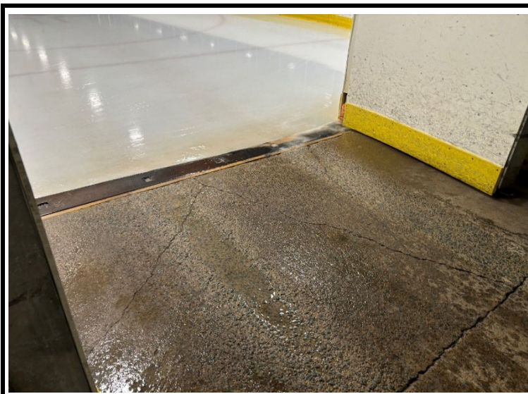
Existing deteriorated concrete slab at Zamboni landing
