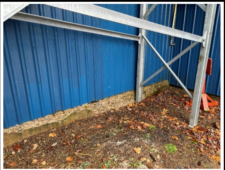
deteriorated concrete at top of foundation wall at rear of building
