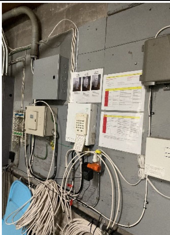
Existing copper backbone telecom service
