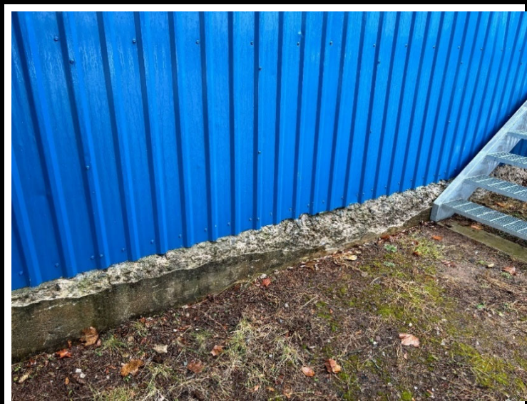
deteriorated concrete at top of foundation wall at rear of building
