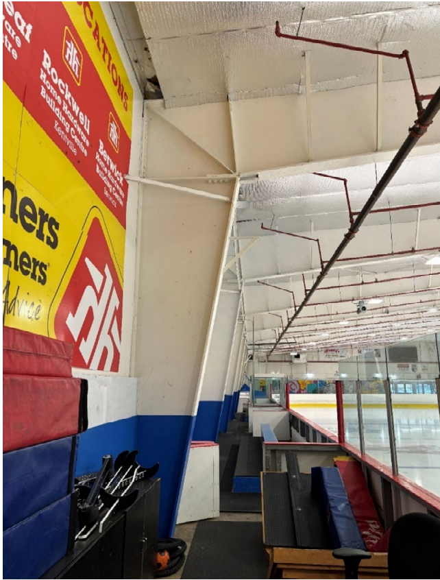
Typical Rigid Frame Column on South Side of Arena
