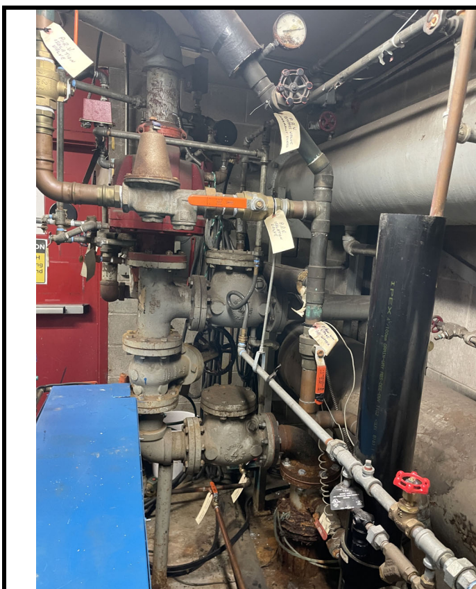
Water service entry to mechanical room
