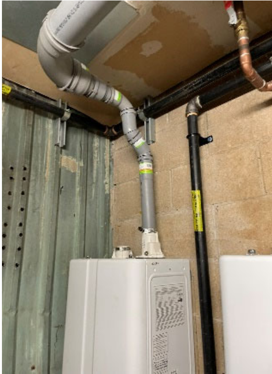
Venting Connections
