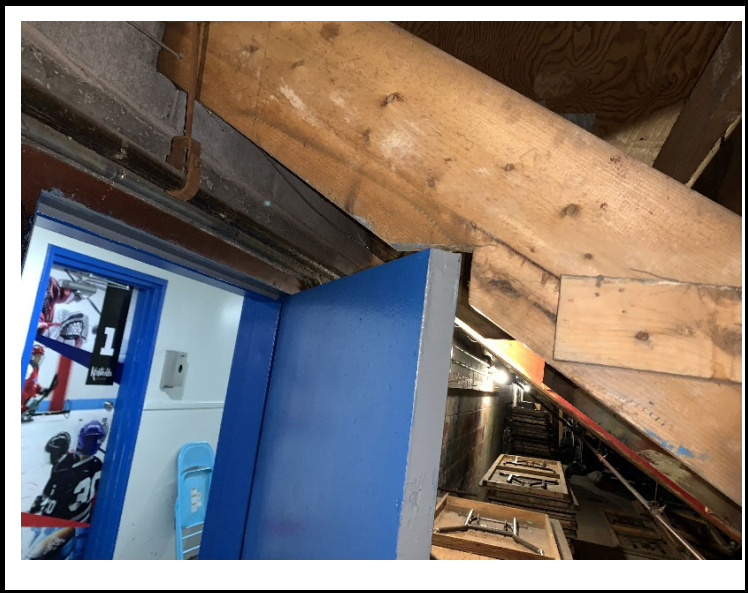
Notches cut into beams under bleachers
