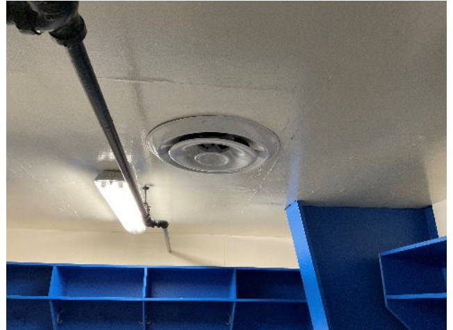
Typical Sprinkler Branch Line
