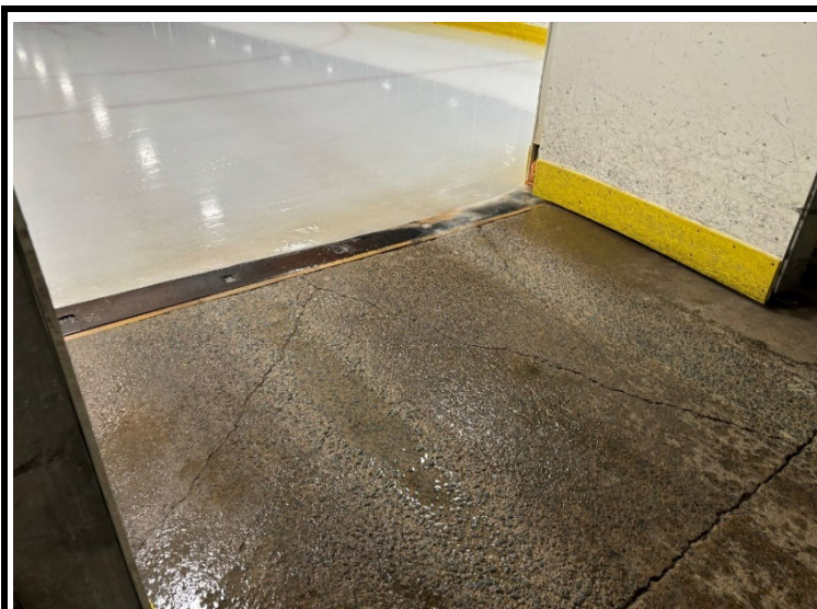
Existing deteriorated concrete slab at Zamboni landing
