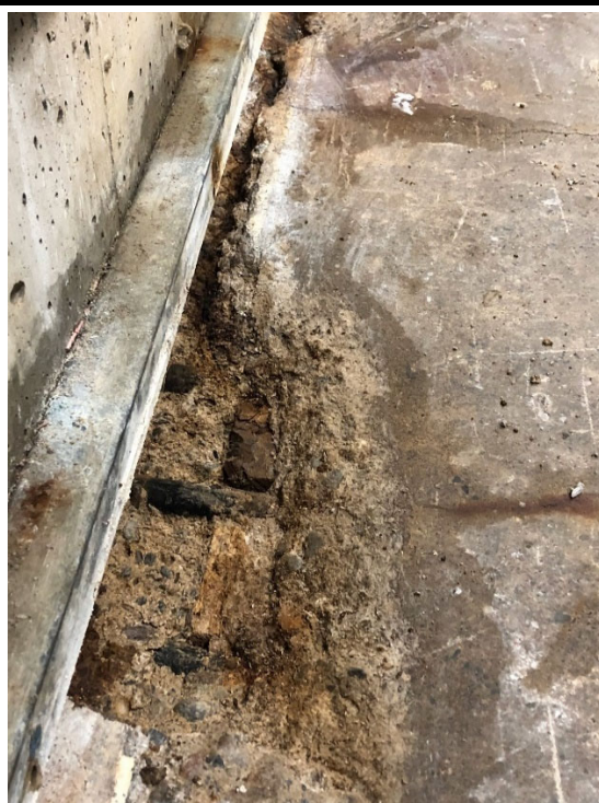
Existing rink slab showing severe spalling & deterioration
