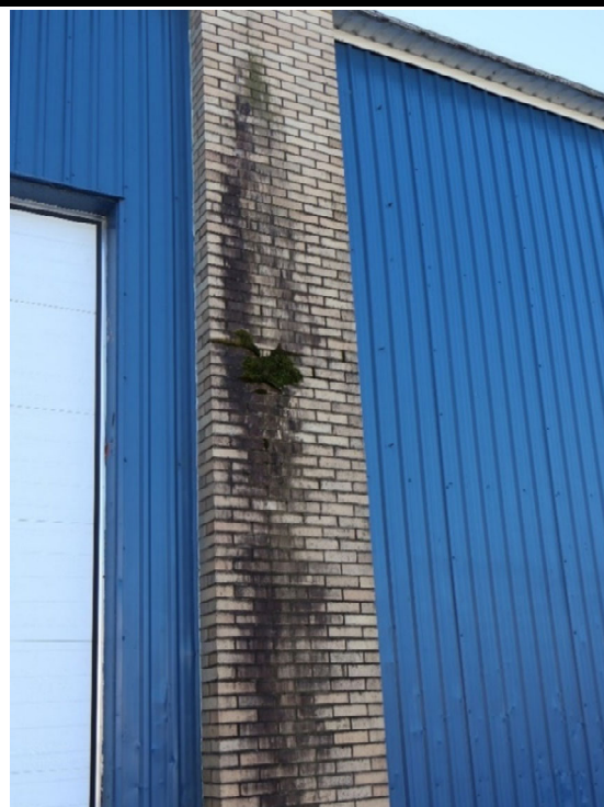
Discolouration of Brick with Mold Growth
