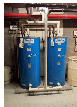
Heat Recover Hot Water Storage Tanks
