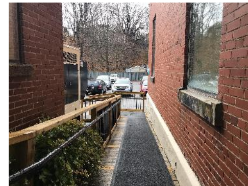
Back Entrance Ramp, Kentville Town Hall
