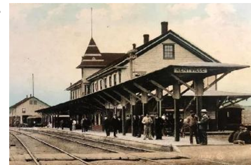
Historical Train Station, Kentville NS
