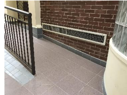
Interior Ramp, Kentville Town Hall
