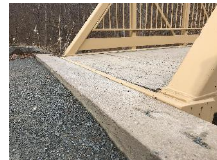
Miner's Marsh, Bridge - Grading Required
