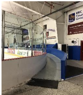
Centennial Arena, Ramp to Separated Accessible Seating
