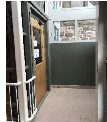
Kentville Library, Elevator
