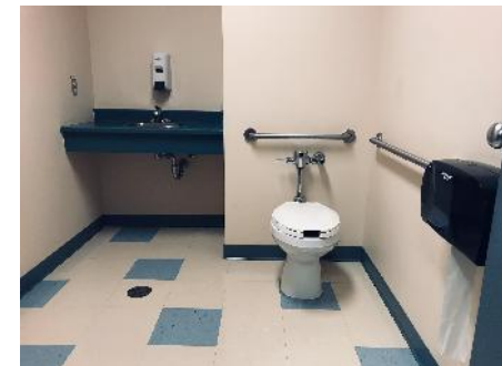
Police Station, Lobby Washrooms
