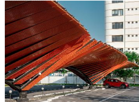
Solar Powered Parking Structures
