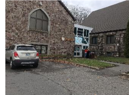
Kentville Library, Accessible Parking not near entrance
