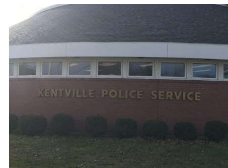
Police Station, Signage
