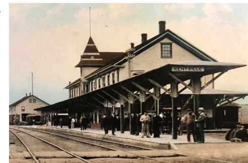
Historical Train Station, Kentville NS
