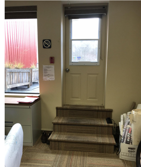
Access to Emergency Exit, Kentville Town Hall
