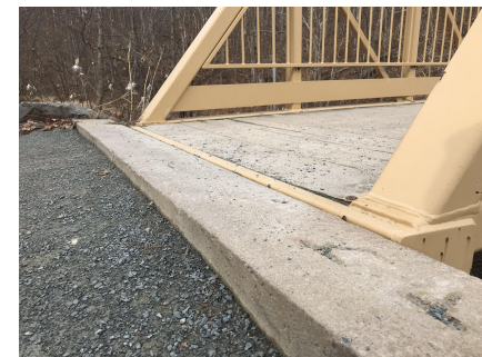
Miner's Marsh, Bridge - Grading Required
