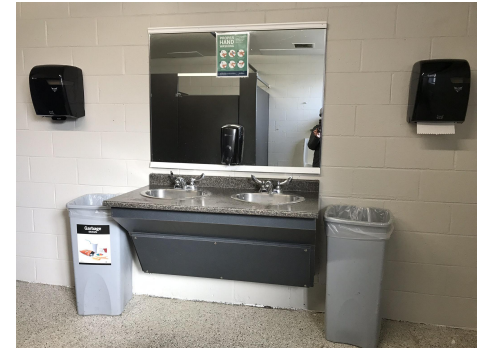
Centennial Arena, Accessible Sink
