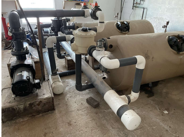
Figure 6 Existing Pool Filtration Room
