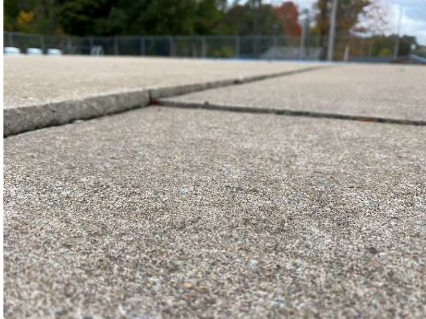
Figure 3 Existing Pool Deck Separation (From Provided Pool Conditions Documentation)
