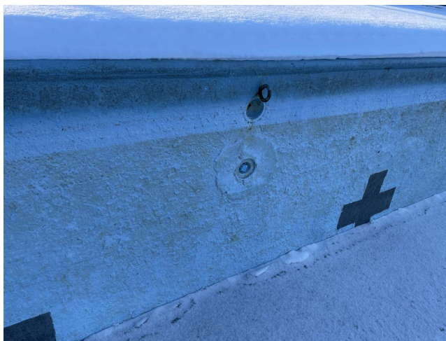
Figure 2 Existing Cup Anchor and Fitting
