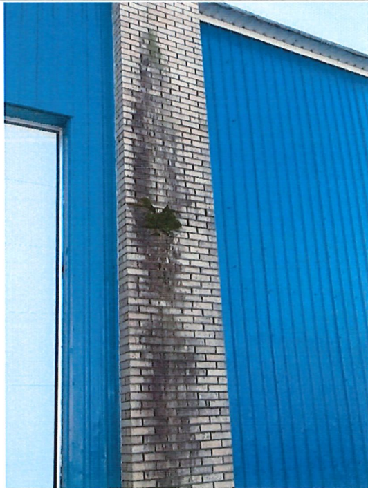
Discolouration of Brick with Mold Growth
