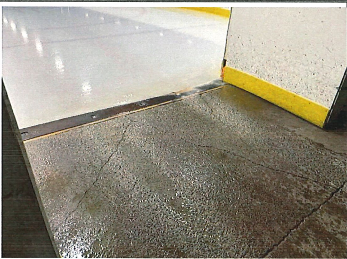
Existing deteriorated concrete slab at Zamboni landing
