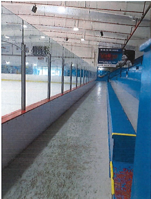
Scratches on painted flooring by the stands
