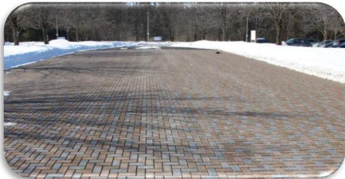
Figure 7-12: Installed Permeable Pavers in Winter (TRCA, 2015)
