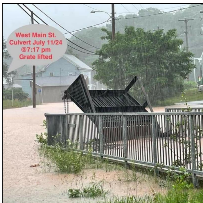
Figure 2-2: Culvert Located at Intersection of West Main Street and Harvest Moon Trail Ditch on July 11, 2024 (Photo Provided by Kentville Resident)
