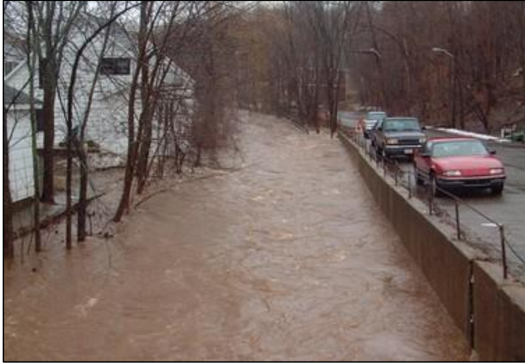
Figure 3-1: Mill Brook Overtopping its Banks March 30, 2003 (Saltwire Network, 2003)
