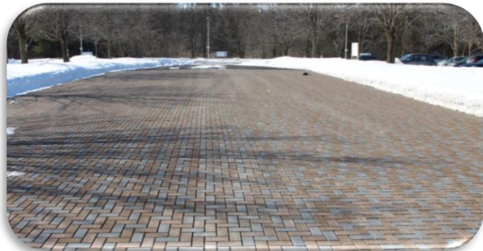
Figure 7-12: Installed Permeable Pavers in Winter (TRCA, 2015)
