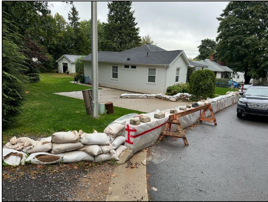
Figure 3-5: Flood Protection Measures at a Residence on Condon Avenue (September 27, 2024)
