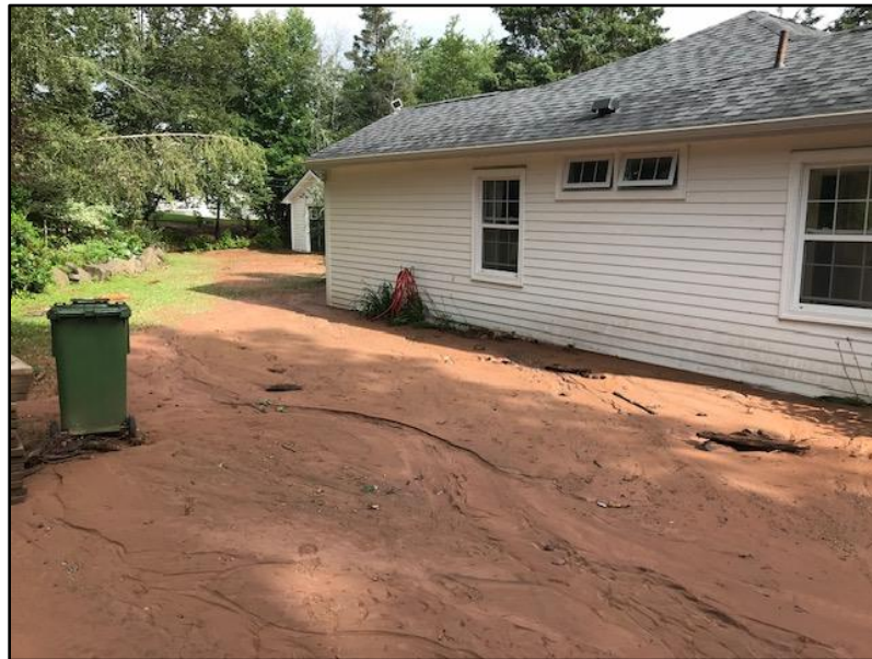
Figure 2-3: Deposited Sediment Covering Yard of a Private Residence on Condon Avenue After a Heavy Rain in 2019 (Photo Provided by Resident of Condon Avenue)
